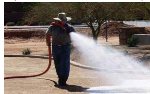
Standard Hose & Pump Hand Spraying
