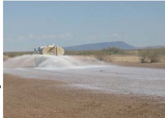
Photos: Environmental Products and Applications Polymers such as Envirotac II are used for long-term coverage or for large areas.
